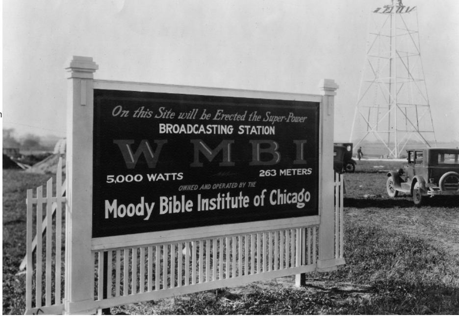
Construction of the WMBI radio station in Addison, Illinois, 1920s.
